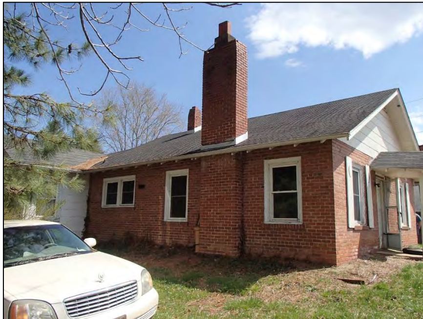
Figure 67: Dumas Family House and Grocery Store, house north elevation
