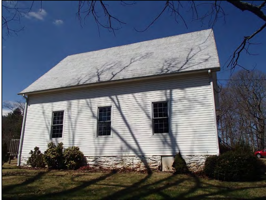
Figure 95: Avery's Creek Christian Church, south elevation
