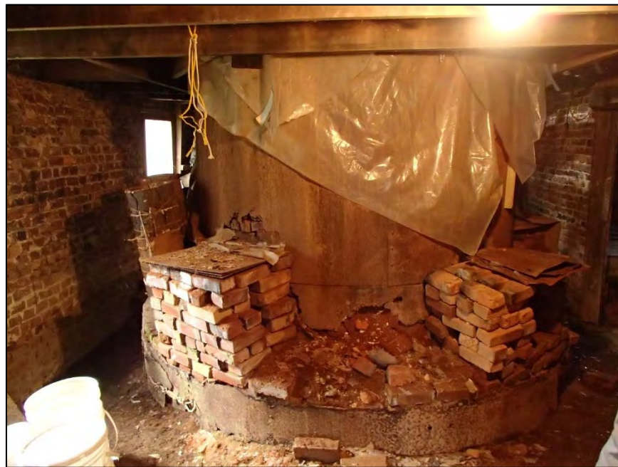
Figure 21: Pisgah Forest Pottery, interior, bottle kiln
