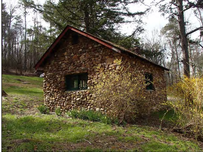
Figure 4: Pisgah Forest Pottery Sales Room, southeast corner
