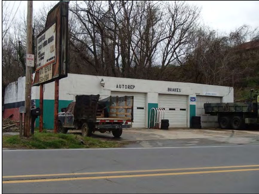
Figure 88: Garage at 880 N.C. Highway 251
