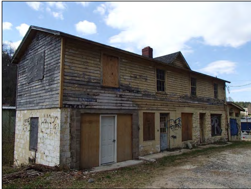
Figure 49: Brooks Store, east elevation
