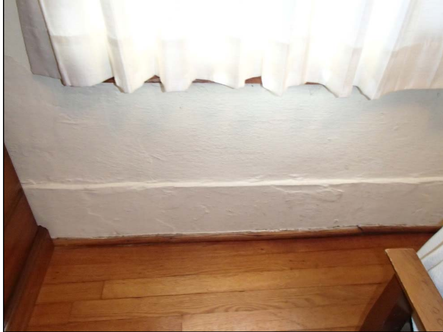
Figure 33: Pisgah Forest Pottery, House, interior, concrete wall with baseboard detail
