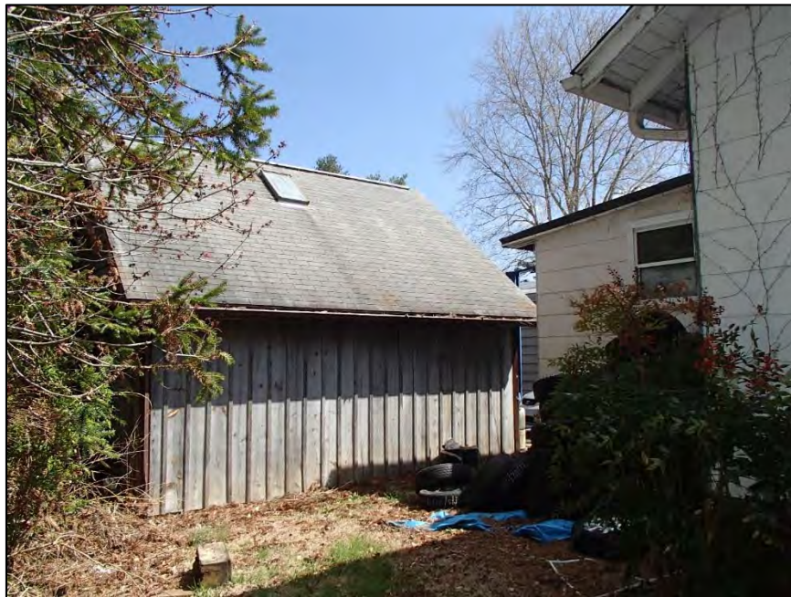
Figure 71: Dumas Family House and Grocery Store, outbuilding
