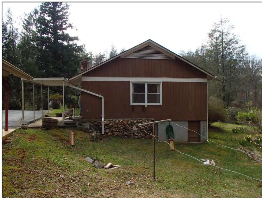
Figure 30: Pisgah Forest Pottery, House, east elevation
