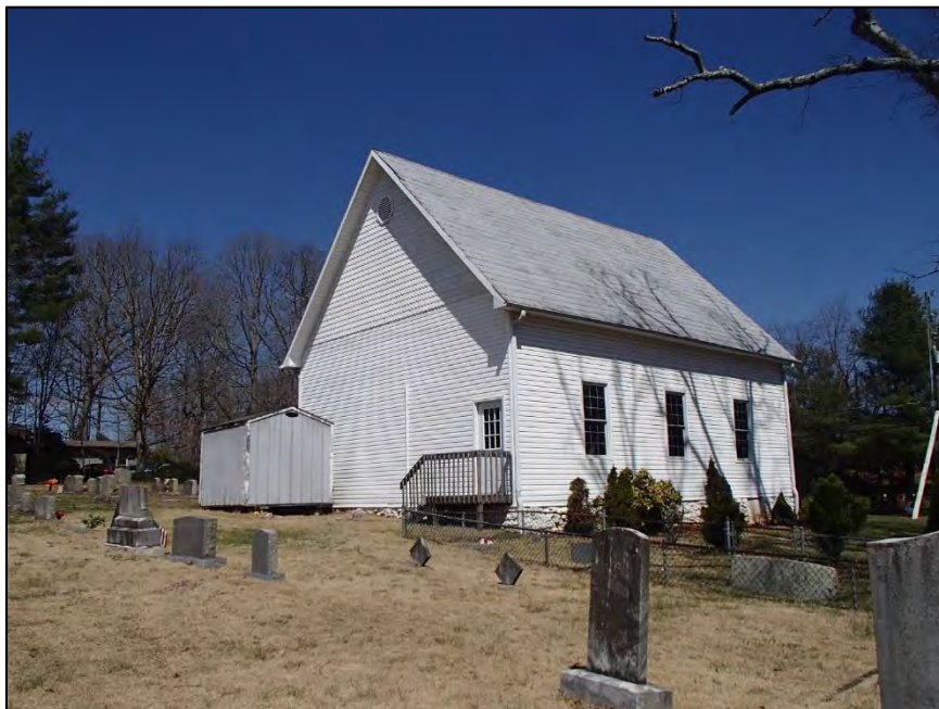
Figure 96: Avery's Creek Christian Church, southwest corner
