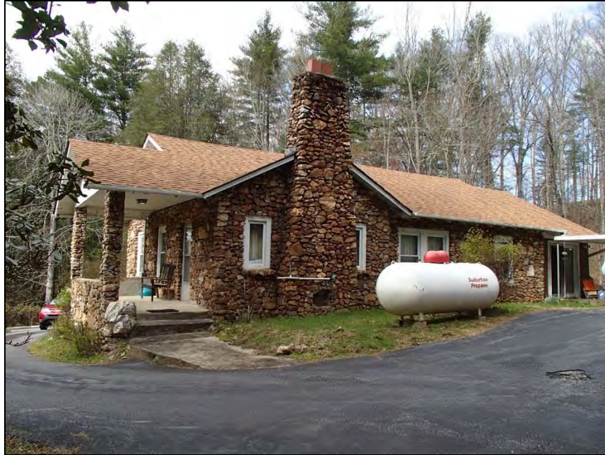
Figure 29: Pisgah Forest Pottery, House, south elevation
