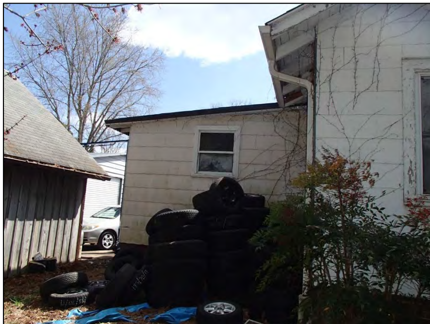
Figure 69: Dumas Family House and Grocery Store, house north elevation detail
