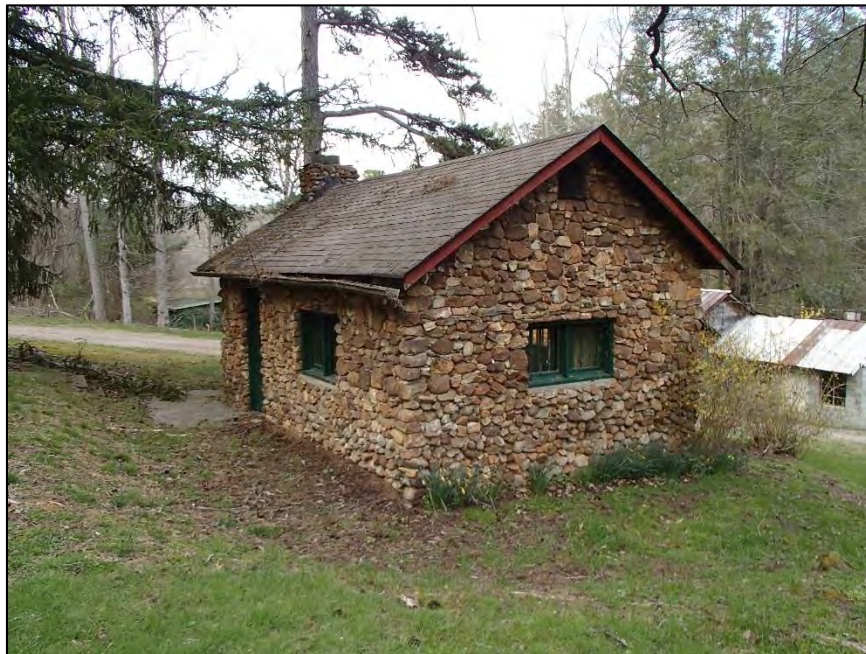
Figure 3: Pisgah Forest Pottery Sales Room, southwest corner
