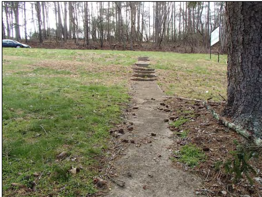
Figure 40: Pisgah Forest Pottery, steps and path from Brevard Road to sales room
