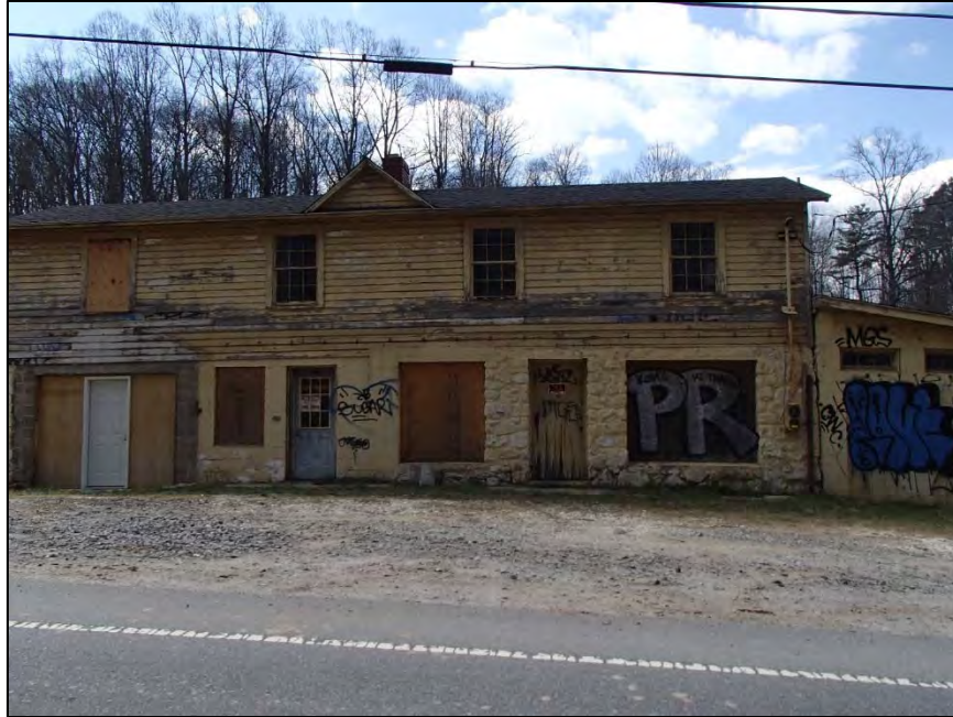
Figure 50: Brooks Store, east elevation
