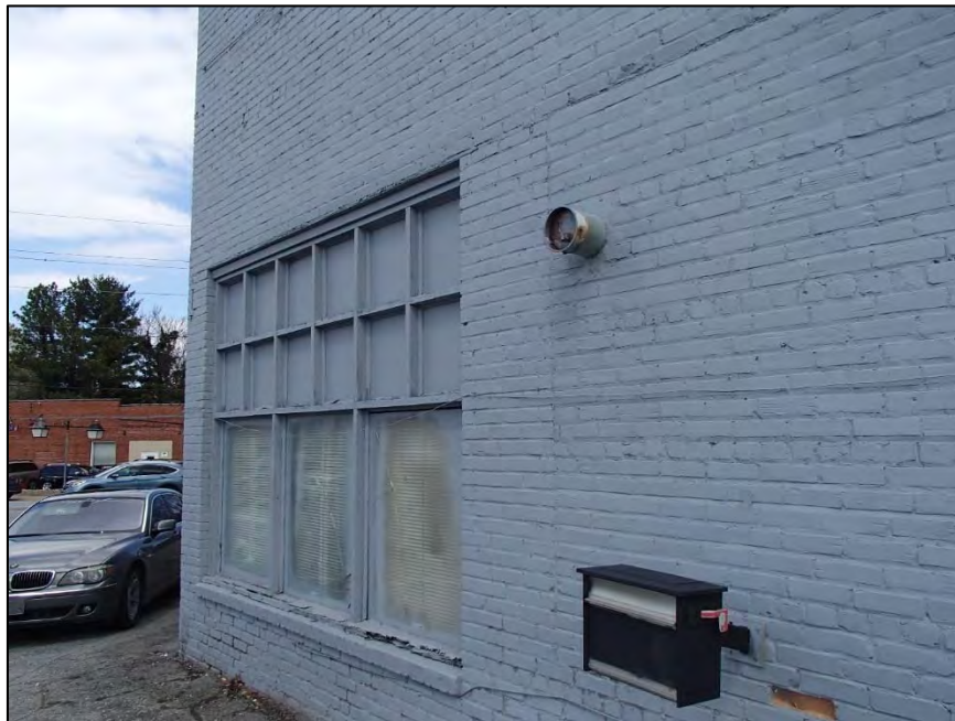
Figure 82: Westhaven Gas Station, west elevation
