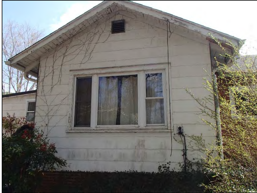
Figure 68: Dumas Family House and Grocery Store, house north elevation detail
