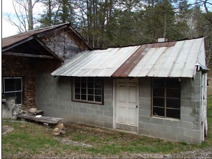
Figure 14: Pisgah Forest Pottery, west elevation of south addition
