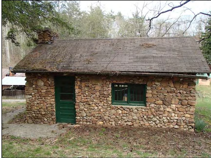
Figure 2: Pisgah Forest Pottery Sales Room, west elevation
