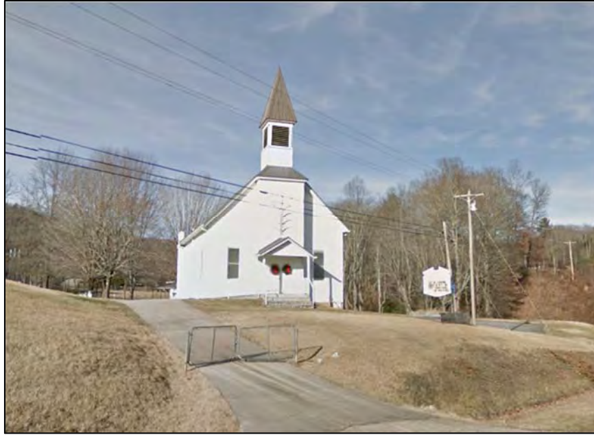
Figure 107: Sandy Mush Methodist Church, 393 Sandy Mush Road (Google Street View image used due to a funeral in progress when the investigator made the site visit)
