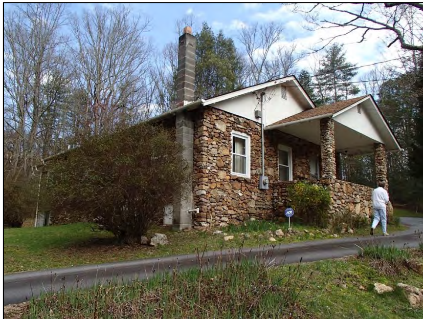
Figure 28: Pisgah Forest Pottery, House, northwest corner
