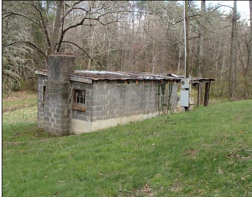
Figure 6: Pisgah Forest Pottery Lone Pine Studio, northeast corner
