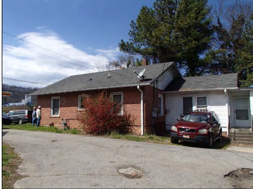
Figure 70: Dumas Family House and Grocery Store, house south elevation
