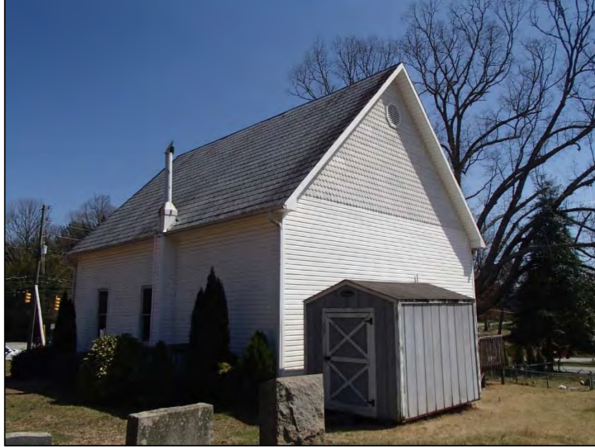
Figure 97: Avery's Creek Christian Church, northwest corner
